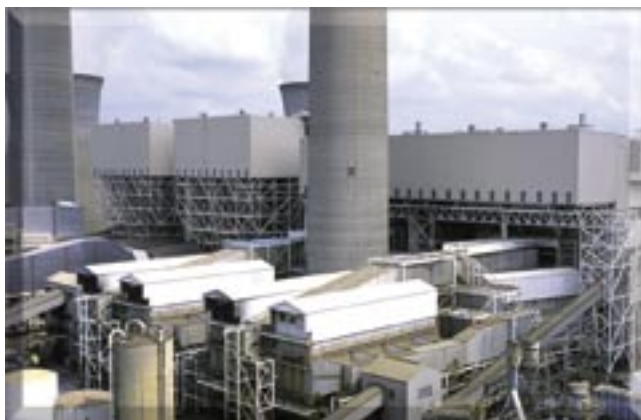
Plant Bowen, Georgia Power Company - Units 1 and 2 SCR's have been operating for 4 ozone seasons. Units 3 and 4 have been operating for 2 ozone seasons.
