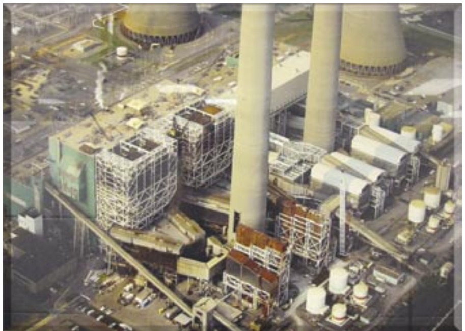
SCR units at Plant Bowen.
